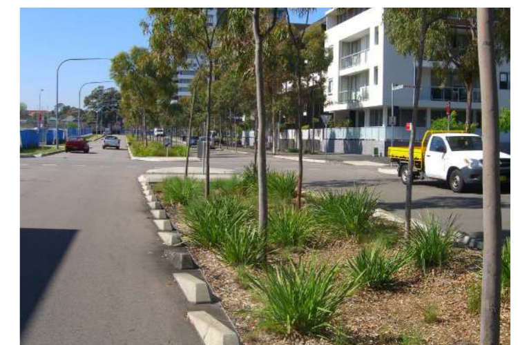
Modified broken kerbs for passive irrigation (Victoria Park, Sydney)
