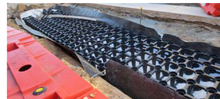
Structural soil cell installation (Featherstone St, Bankstown)
